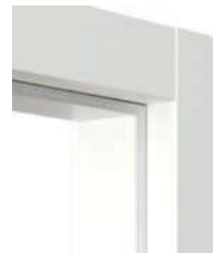
Main beam recessed. Door frame finished with UV acrylic paint.
