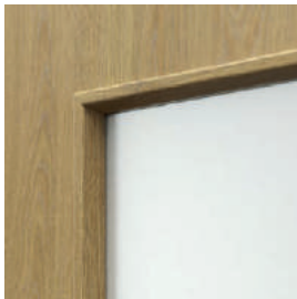
a glazing bead with a glass panel
