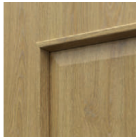
a glazing bead with a raised panel
