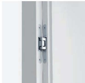
Door frame corner from hinges side
