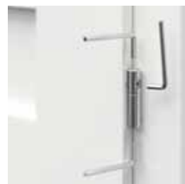
adjustment of 3D adjustable barrel hinges
