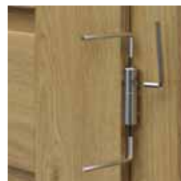
adjustment of 3D adjustable barrel hinges
