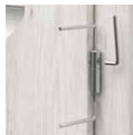
adjustment of 3D adjustable barrel hinges
